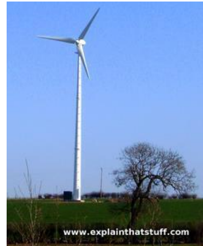
Photo: Making clean, renewable energy from the wind. Each of these turbines contains an electricity generator in the top section, just behind the spinning rotors.
